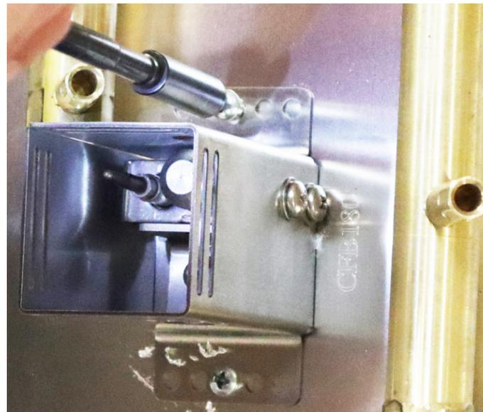
Photo 5: Securing the Pilot to the Plate/Pan
