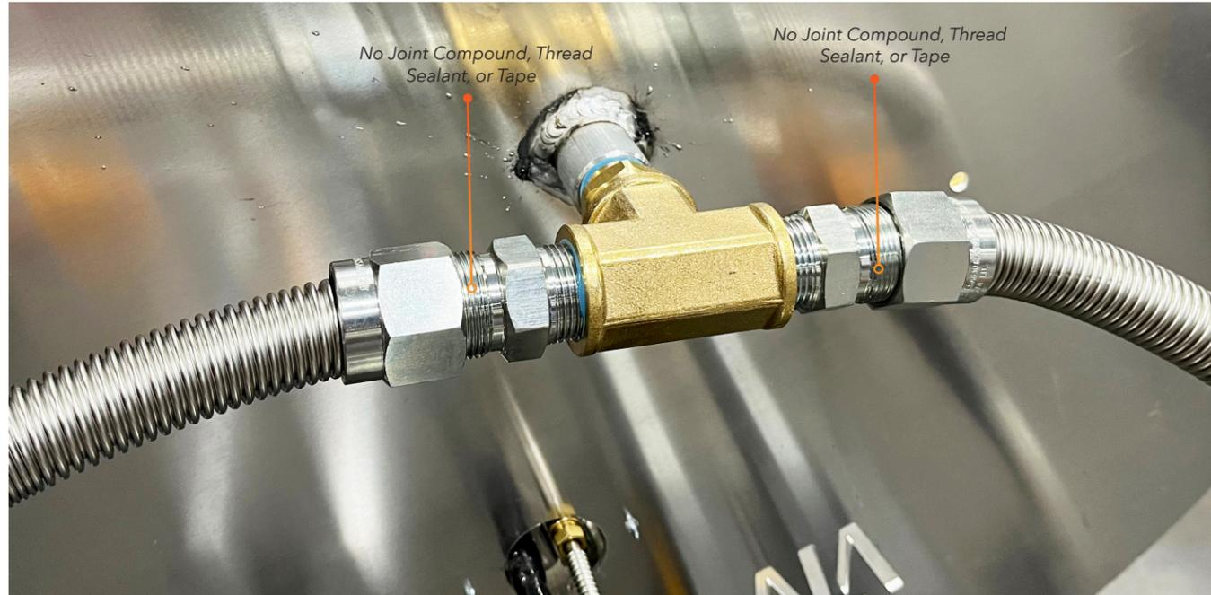
Photo 20: Connecting the Flex Lines
