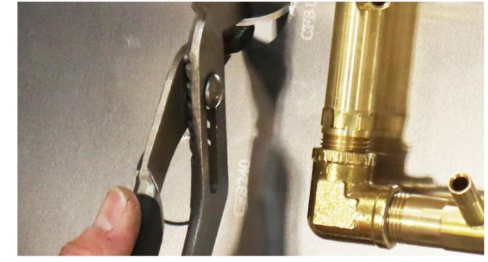
Photo 2: Breaking the Knockouts
