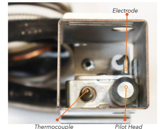
Photo 3b: Top-Down View of Pilot Assembly
